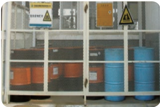
Storage of used mineral oil at Axle & Transmission Company
