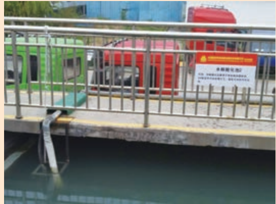
● Upgrading of waste water treatment facility for hydrolysis acidification pool
