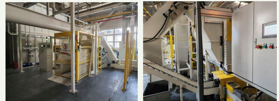
Ji'nan Transmission Plant has reconstructed its iron filings pond
